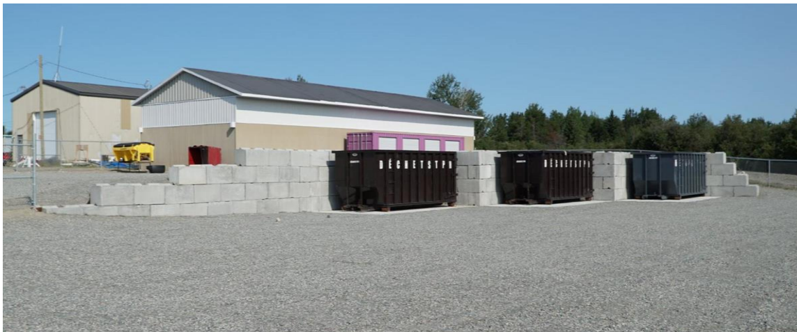
Figure 10: Wood, metal and bulky waste container, Pikogan ecocenter
